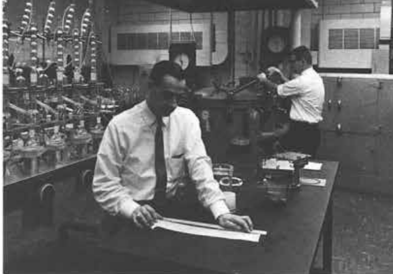
C. J. Spiegl prepares packaging materials for extractability studies while A. M. Palmer adjusts the steam autoclave used for experiments at sterilization temperatures.
