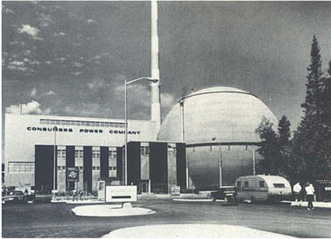
Consumers Power Company's Big Rock Point Nuclear Power Plant near Charlevoix has been in operation since 1962, first as a research and development facility and later as a power producer. The plant's boiling water reactor and turbogenerator unit are rated at 75,000 kw.
