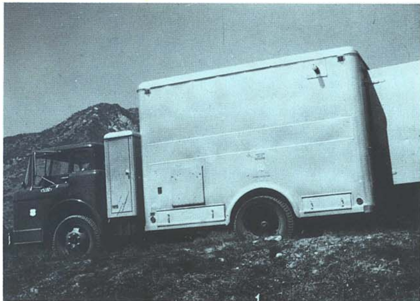
This is one of three mobile spectrographic units operated by U.S. Geological Survey for extensive mineral evaluation in primitive areas of the western United States. A crew of four may analyze as many as 120 samples per day for 30 elements.
