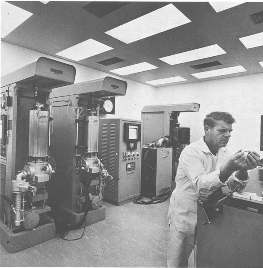
Spectroscopist F. R. Fucek preparing to excite a steel sample in the emission spectrograph.
